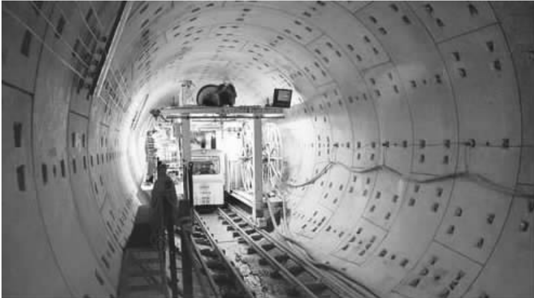
Figure 1.2 A Metro Tunnel
